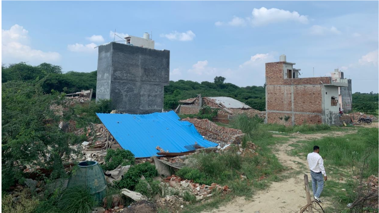
Figure 1: Aftermath of state violence and demolitions in agrarian Delhi (Image Credits: Sahil Sasidharan, 2023)
